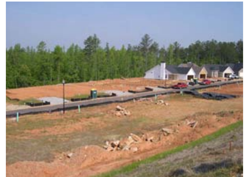
Open-wall panel houses under construction in Newman, Georgia
