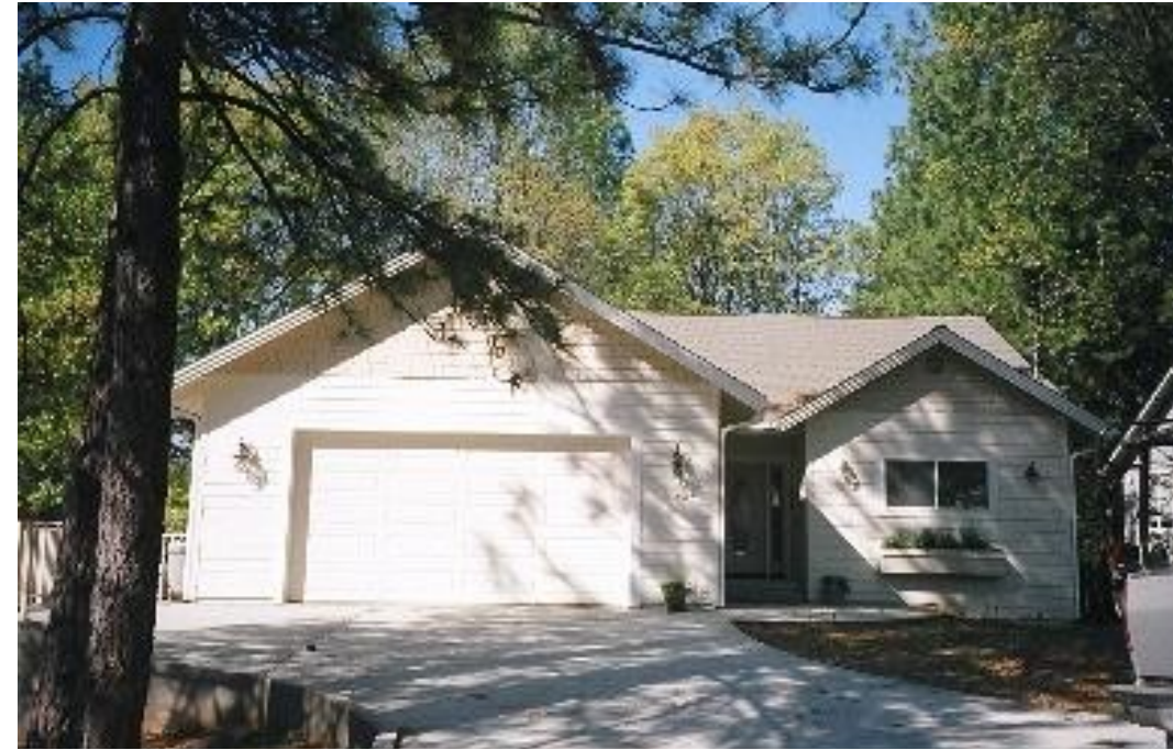
Finished panelized home in Northern California
