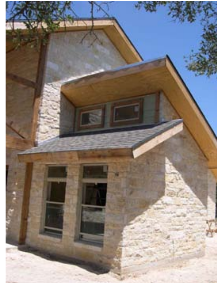
Panelized house with stone cladding under construction in Texas
