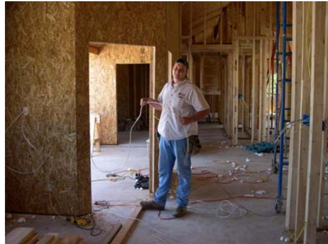
Electrician wiring a structural insulated panel house in Texas
