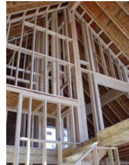
SIP house with stick construction infill
