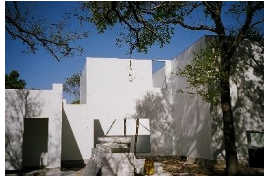
Metal structural insulated panel house under construction in Florida
