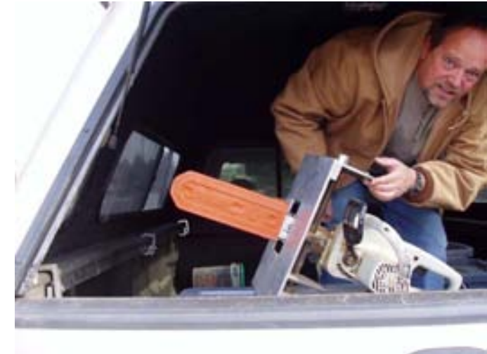
Getting ready to trim a SIP, an on-site operation in Colorado
