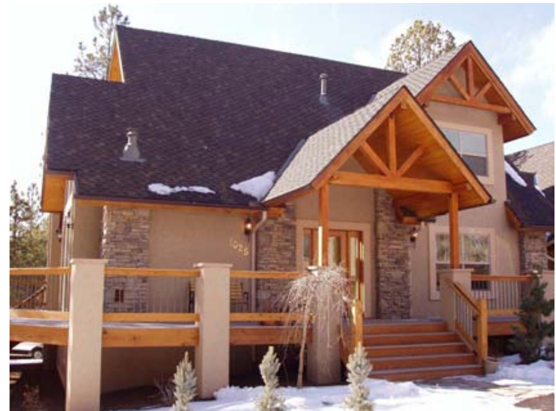
Completed wood-framed panelized home in Colorado
