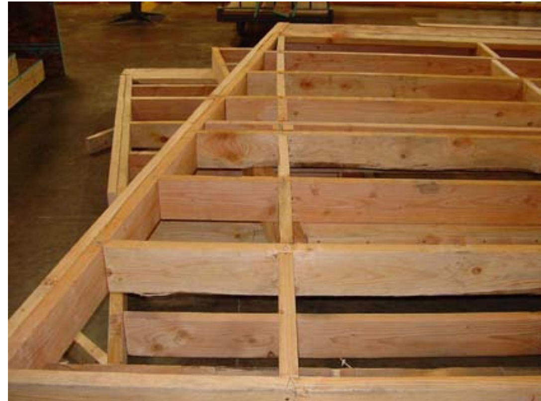
Open-wall panels stacked in a factory during manufacturing in California
