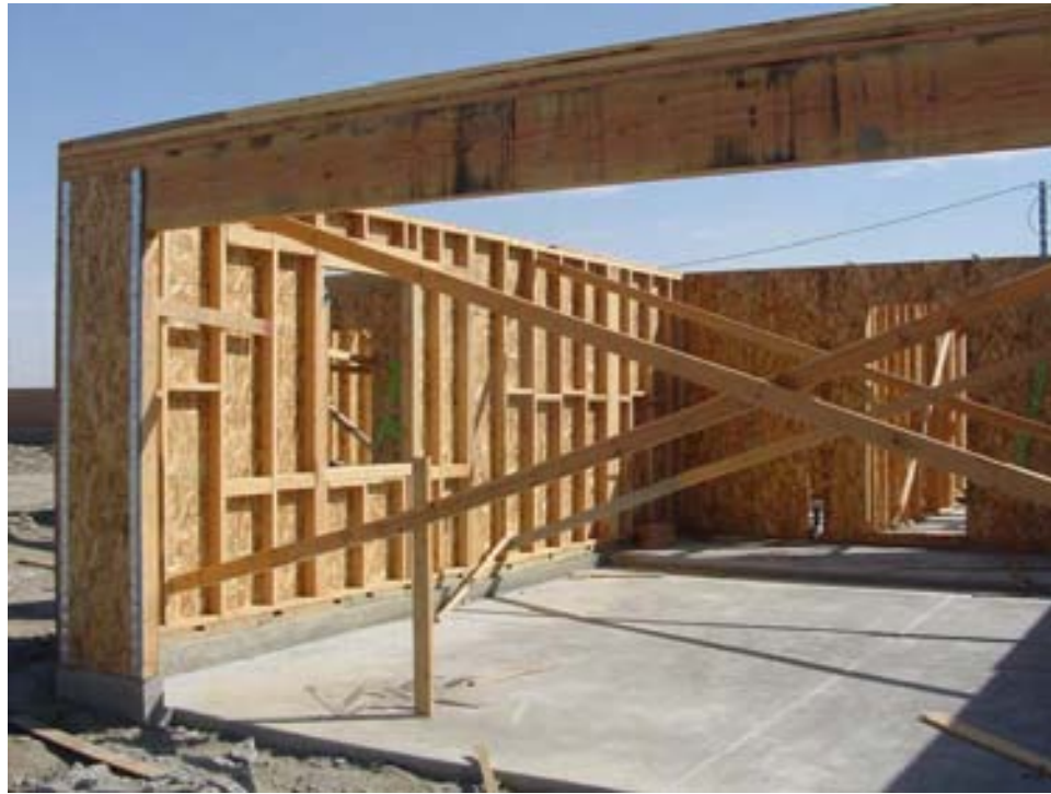
Open-wall wood-framed panel system used in Coachella, California
