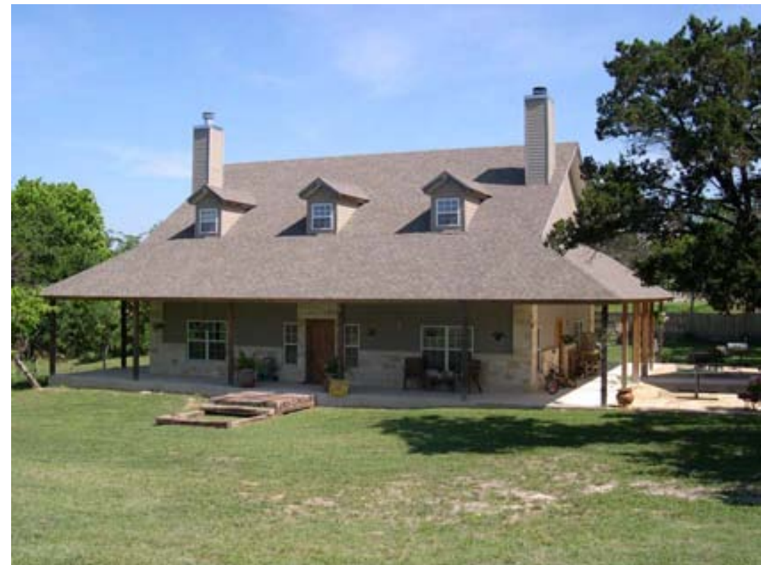
Builder’s own panelized home in Kerrville, Texas
