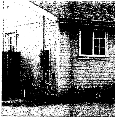
Exterior meter base installed after the home was installed, cluttering the side of the house.
